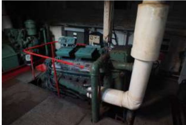
Port main propulsion unit.
