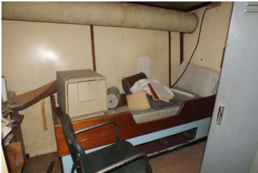
Aft starboard stateroom.
